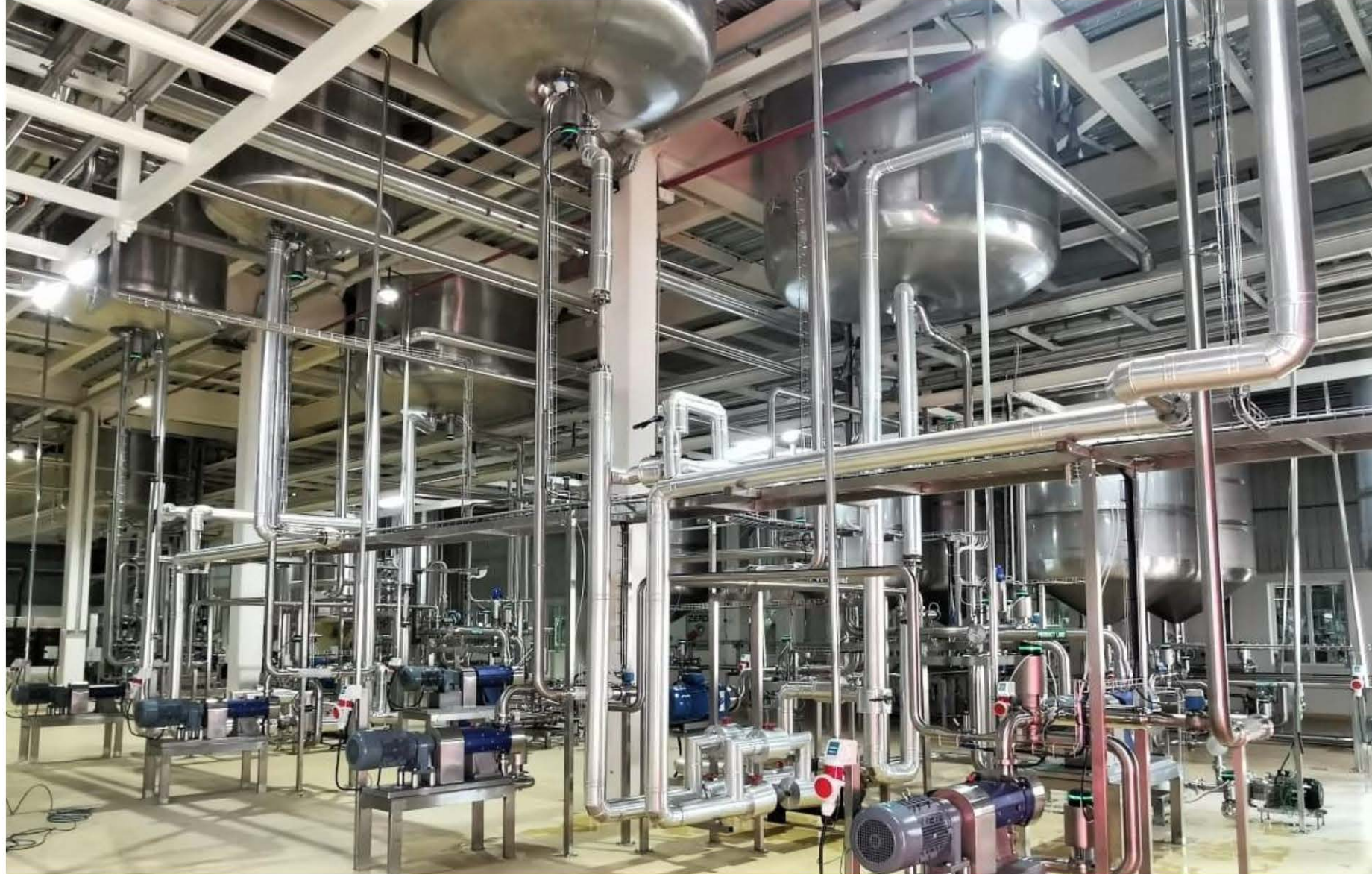
Hyderabad | Liquid Detergent Plant
