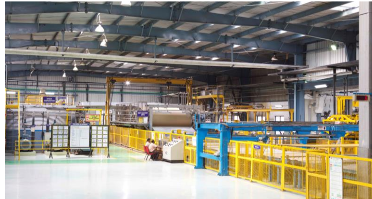
Mysore factory - 100% green electrification
