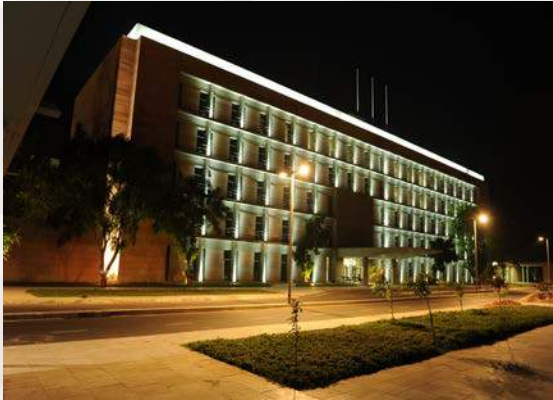
Swarnim Sankul 1 & 2 Construction and interior work
