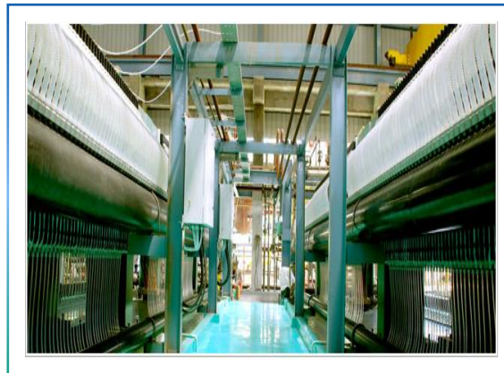
Caustic Soda manufacturing, Karaikal, Puducherry
