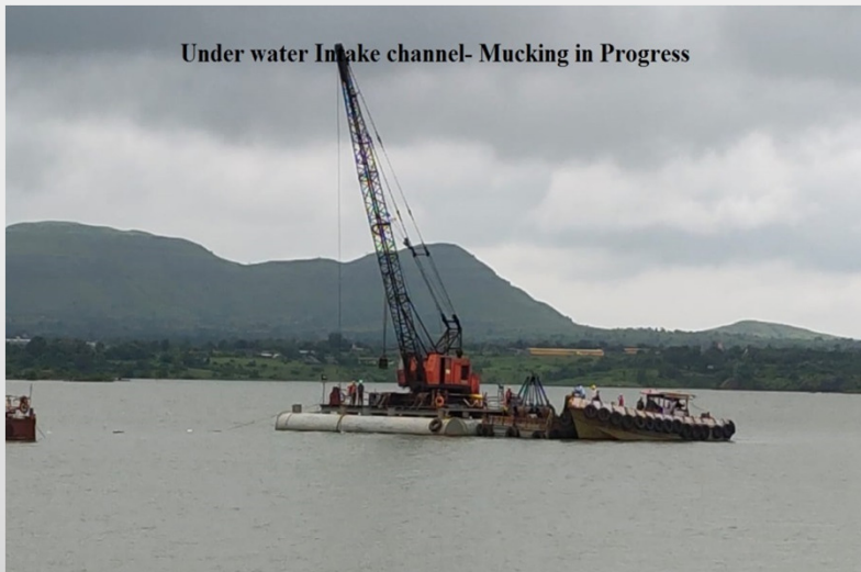
Irrigation Work in progress, Bhama, Pune
