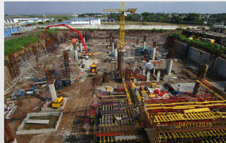
Pune Airport Modernisation – In Progress
