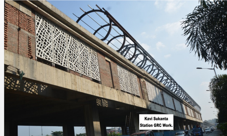
RVNL Station, Kolkata - In Progress
