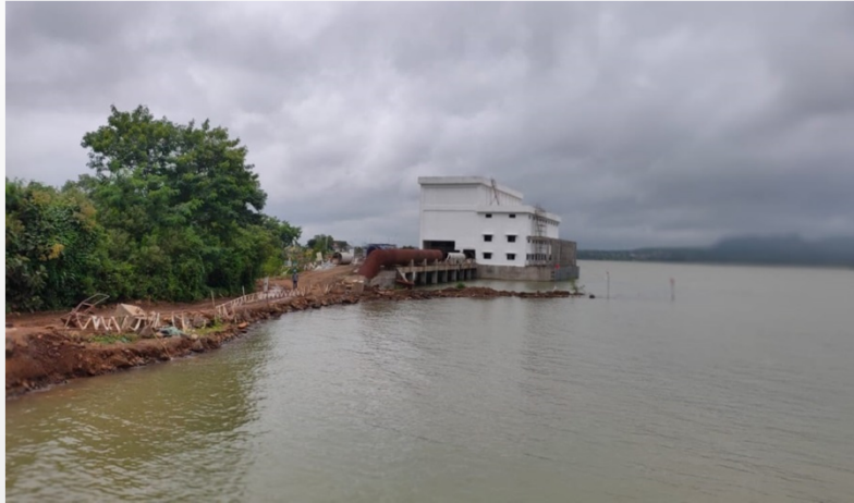
Bhama Ashed Water Supply Project
