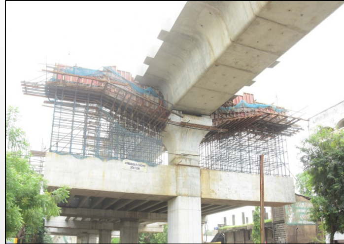
Nagpur Metro Project – In Progress
