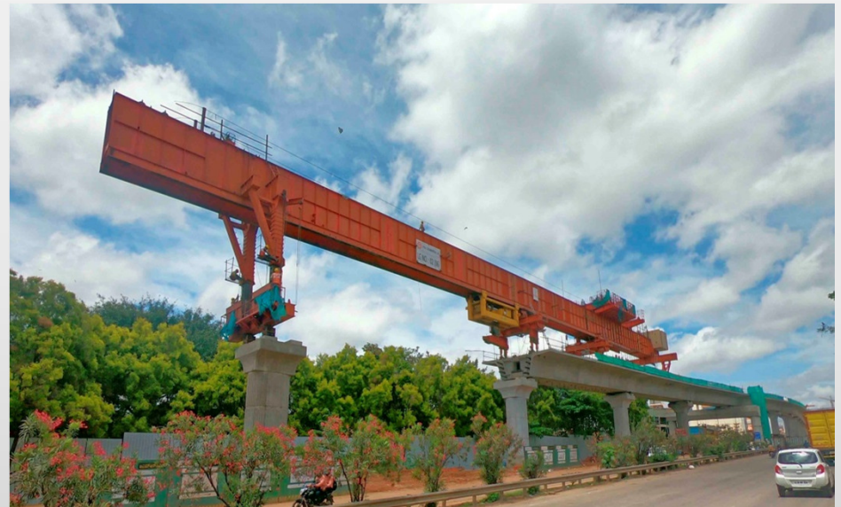
Bangalore Metro Erection Work in Progress
