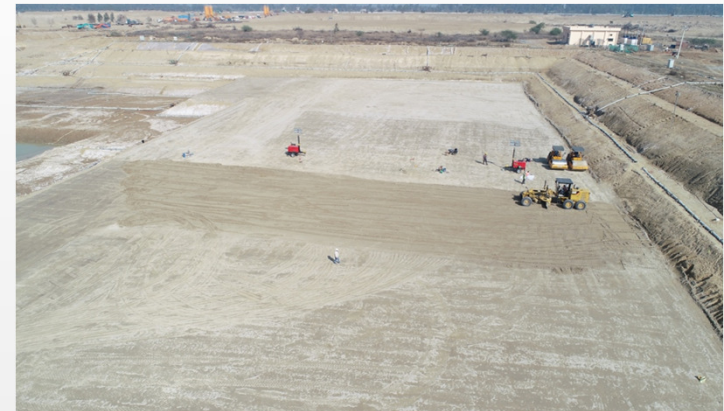
Ground Stabilisation work for Nuclear Power Corporation
