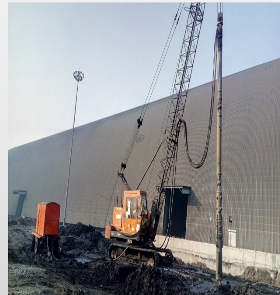
Stone Column Work at Jindal Steel
