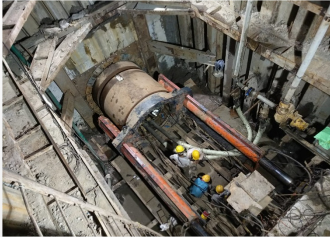
Micro Tunnelling Project, Kolkata
