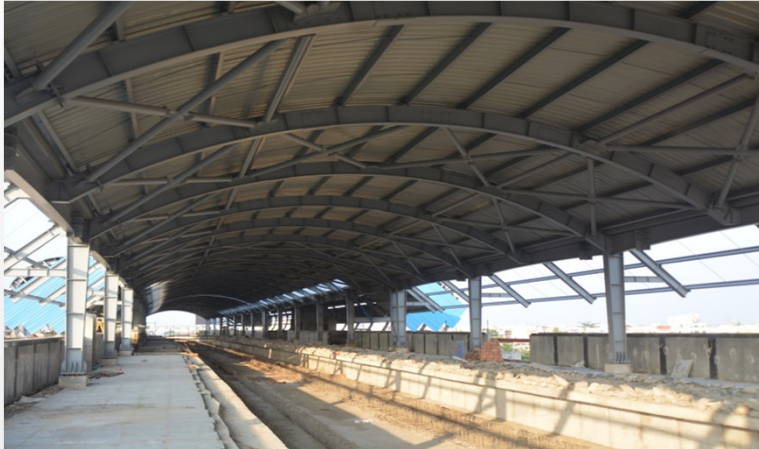
RVNL Station, Kolkata – In Progress
