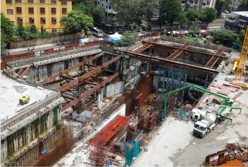
Underground Siddhivinayak Metro Station under Construction
