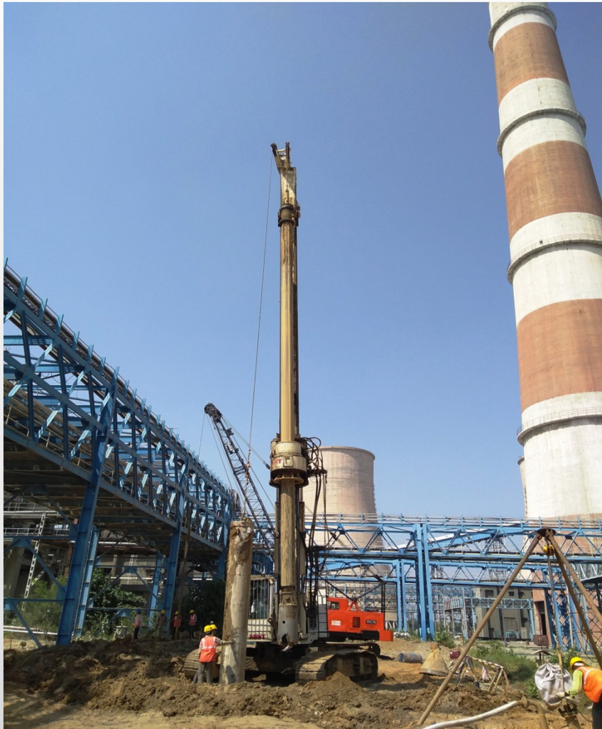
Piling at GE Power Project, Jhajjar
