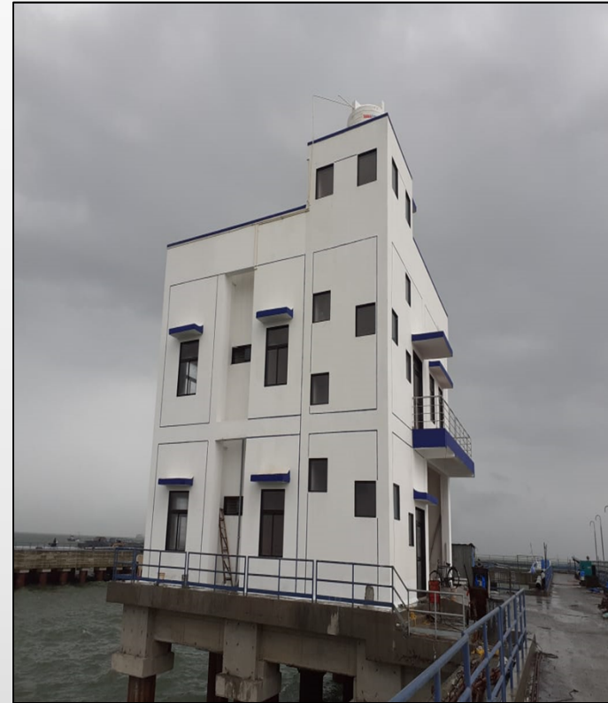
Control Room Building on a Jetty Platform, MbPT
