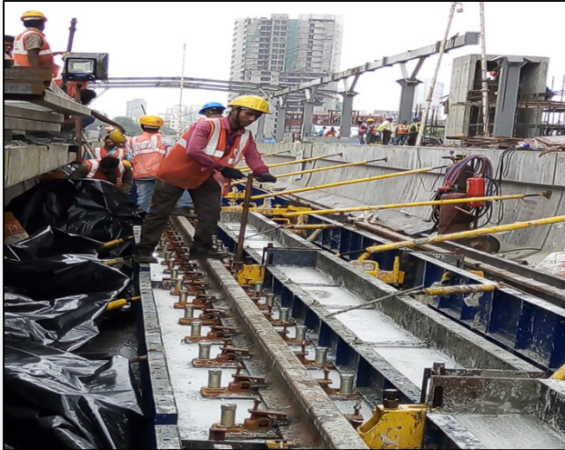
Trackwork Progress for MMRDA, Mumbai
