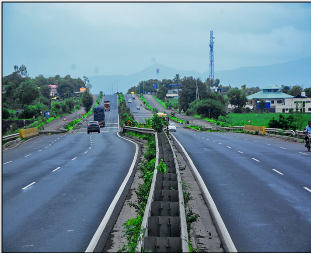
Pune Satara Road Project
