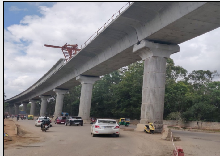
Bangalore Metro – In Progress
