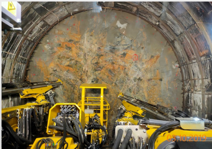
Drill & Blast Tunnel for Indian Railways
