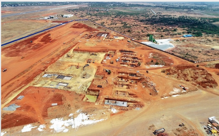
Trichy Airport Modernisation
