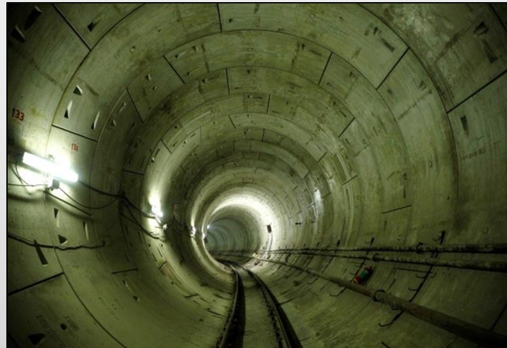
TBM Tunnel, Mumbai
