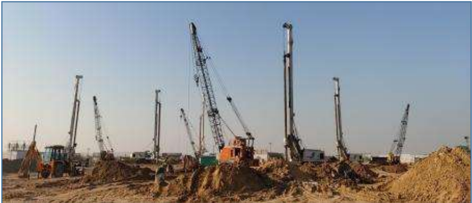
Piling work at Barmer project in Rajasthan
