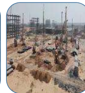
FOUNDATION AND SPECIALIST ENGINEERING
