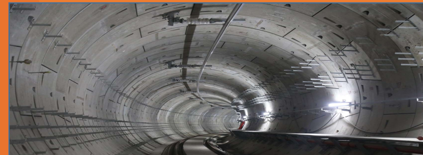
Mumbai Metro underground tunnel in Maharashtra
