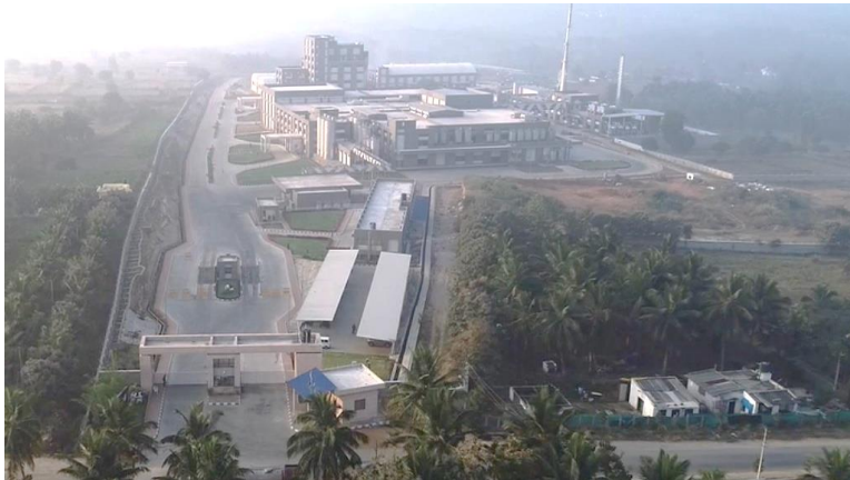
BANGALORE MILK UNION DAIRY PLANT AT KANAKPURA, KARNATAKA
