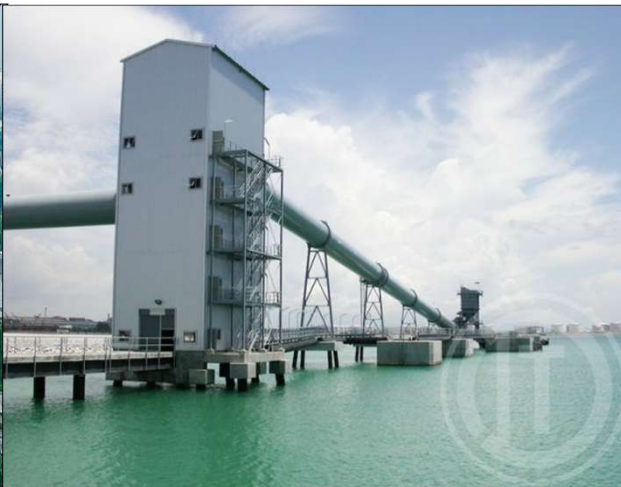
COCO Coal Handling System
