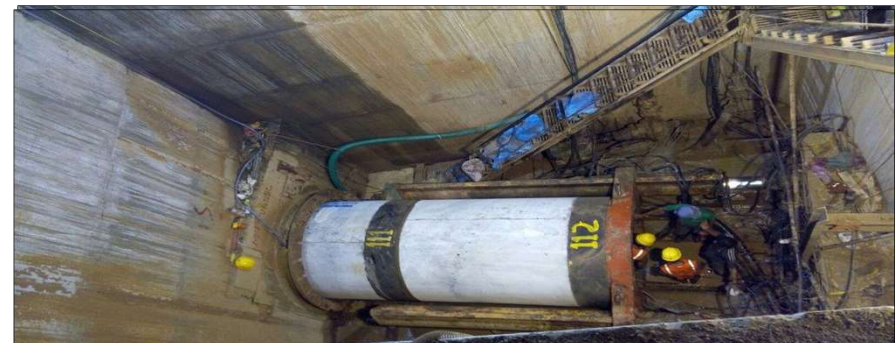
VMSS – Micro Tunneling Vadodara
