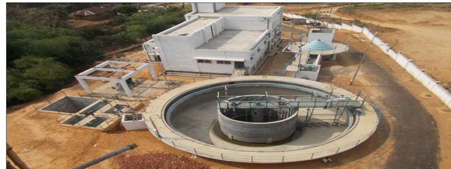
Agartala WTP project
