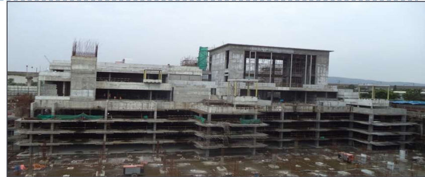
Civil Works Wadala
