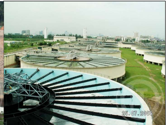
Bang Khen Water Treatment Plant , Bangkok
