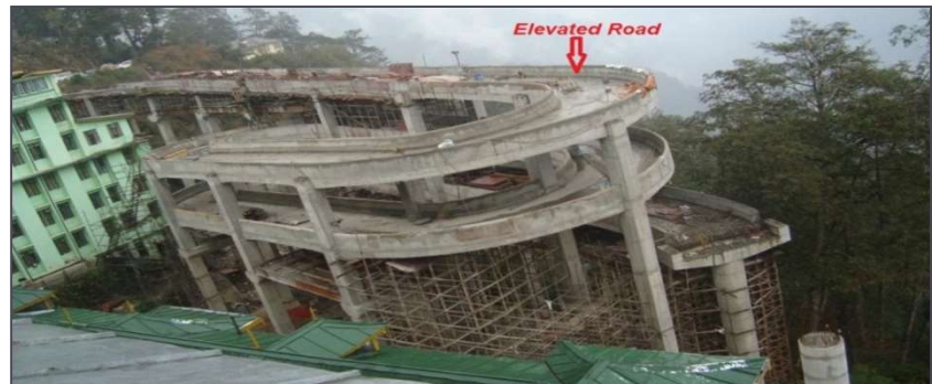
Piling & Civil Arctech, Gangtok
