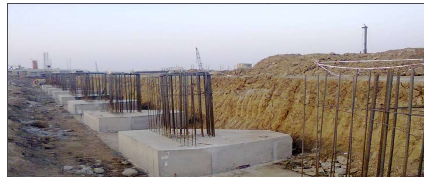
Foundation BASF, Dahej
