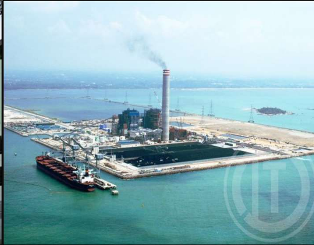
BLCP 2 x 700 Mw Coal Fired Power Plant (Civil Works)
