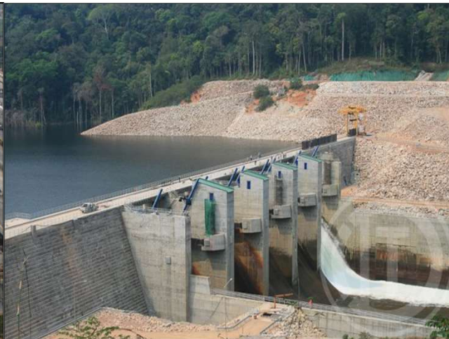
Nam Theun 2 Hydroelectric Project Contract CW1 and CW3
