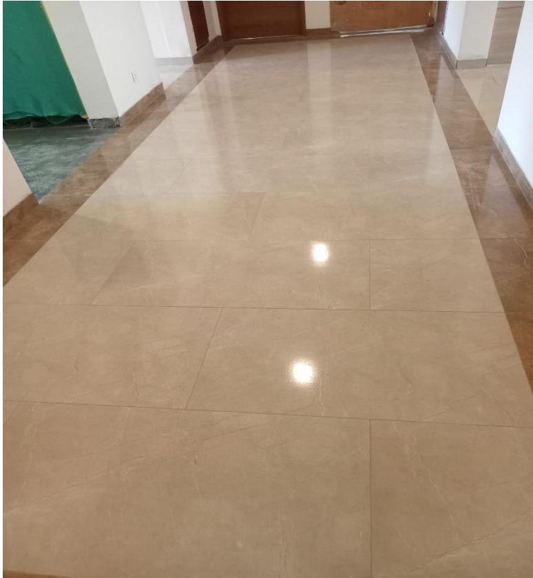
Common Area Flooring
