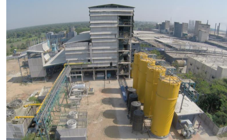
Multiple Effect Evaporator Plant (MEEP)
