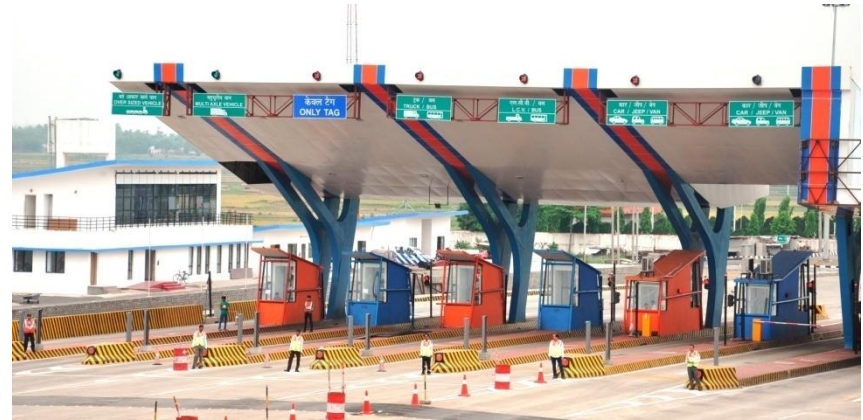
Package 3 Toll Plaza at Km 206
