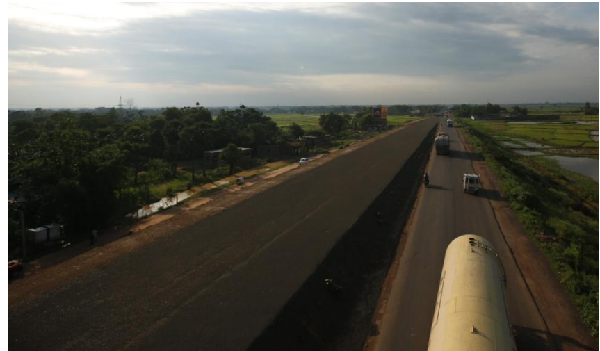
Construction underway at Package 4
