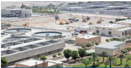
Water Treatment Plant, Doha
