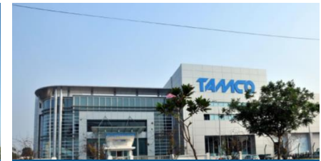
MV Switchgear Factory, Malaysia
