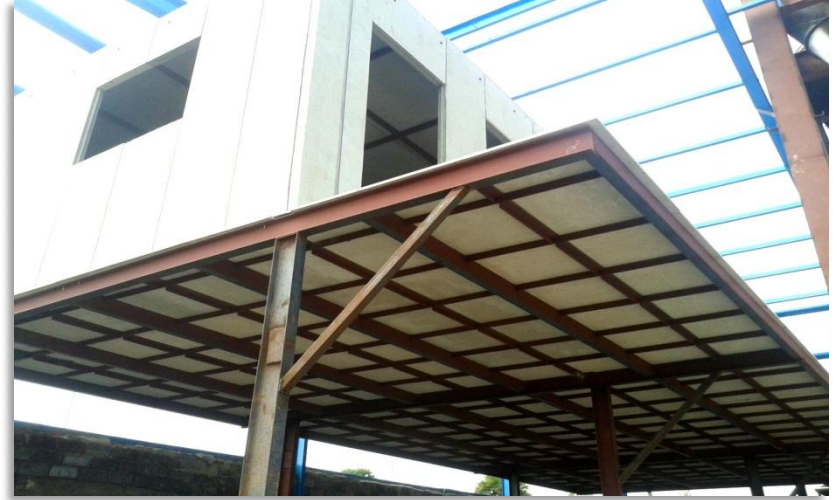
Mezzanine flooring - (V-Board)
