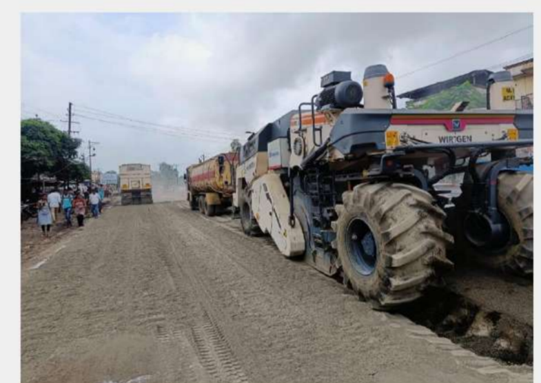
Pulverization of soil with Recycler
