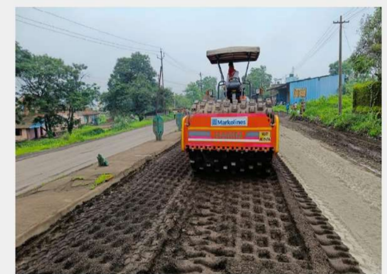
Compaction by Pad Foot Roller
