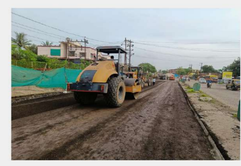
Compaction by Soil Compactor
