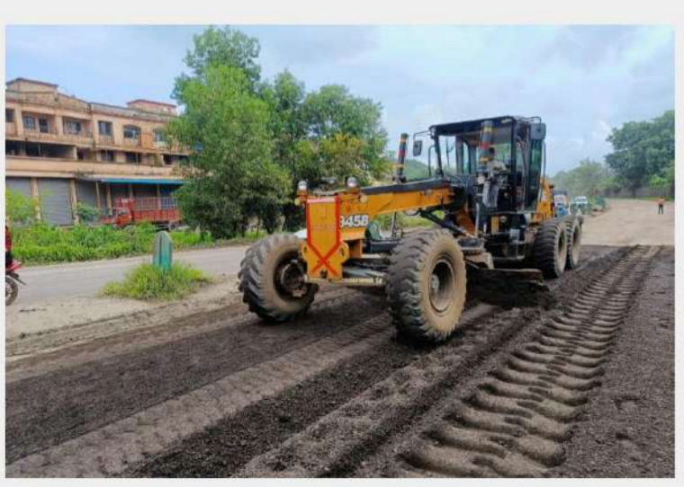
Grading & Profiling with motor Grader
