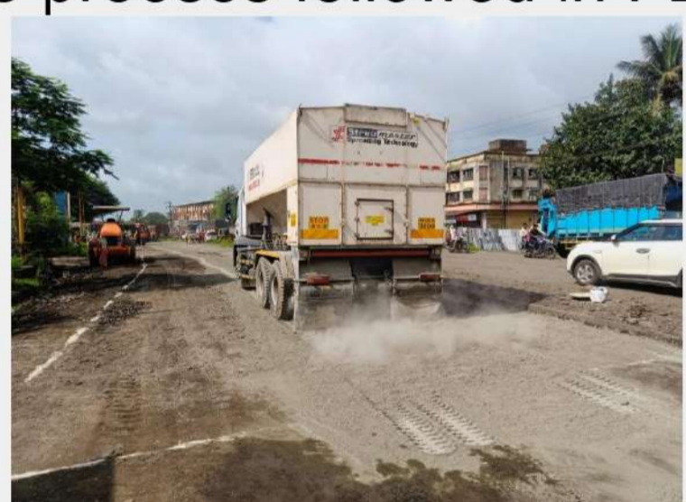
Cement Spreading by Microprocessor Controlled Spreader Truck
