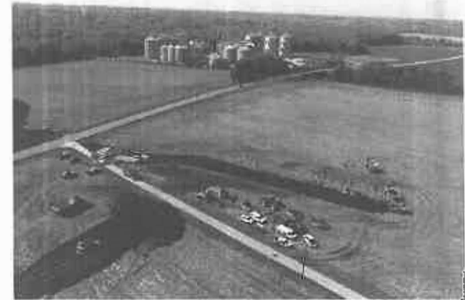
Beginning to break ground in Guthrie, Kentucky
