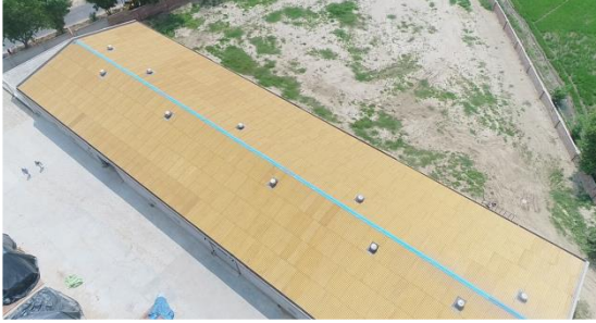
Everest Super Manufacturing Plant, Gidderbaha, Punjab
