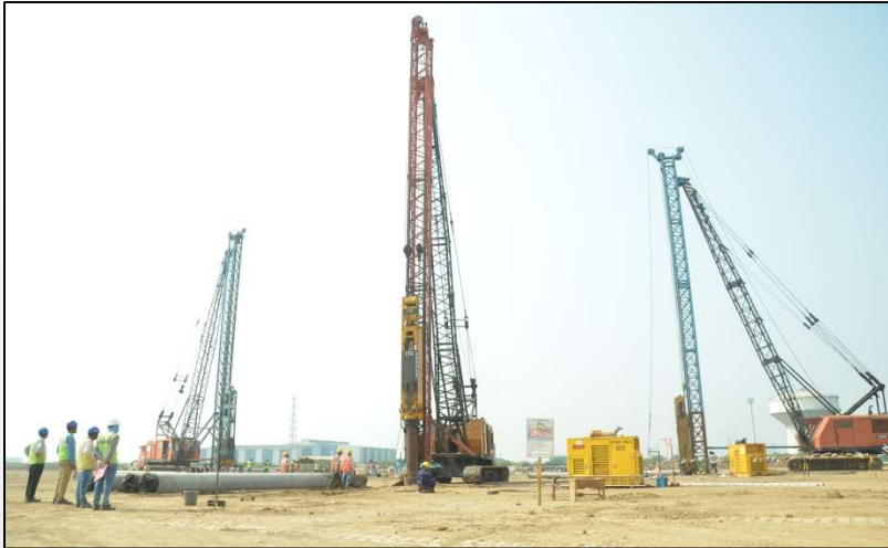
CINDA, Dahej Spun Piles
