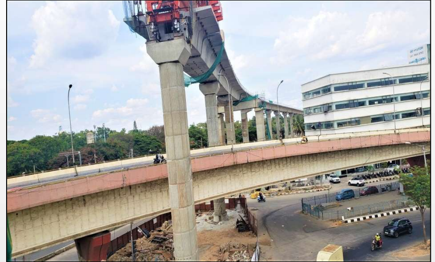
LG Crossing Over Existing Flyover, BMRCL Project
