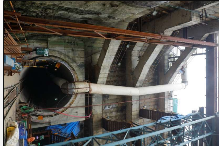
Underground Tunneling at Siddhivinayak, Mumbai
