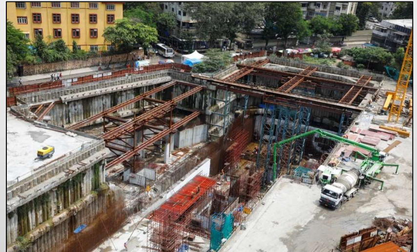
Underground Siddhivinayak Metro Station under Construction
