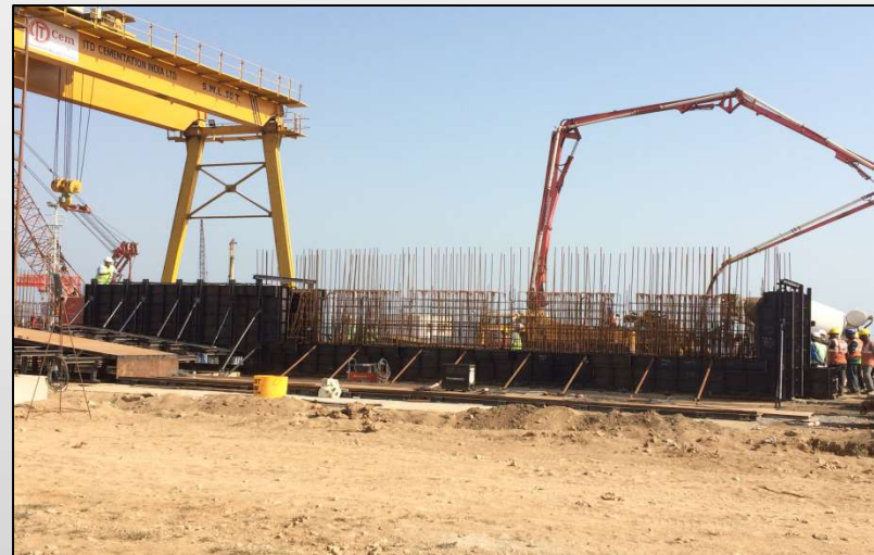
Chhara Port – In Progress
