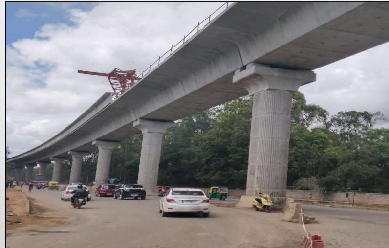
Bangalore Metro – In Progress
