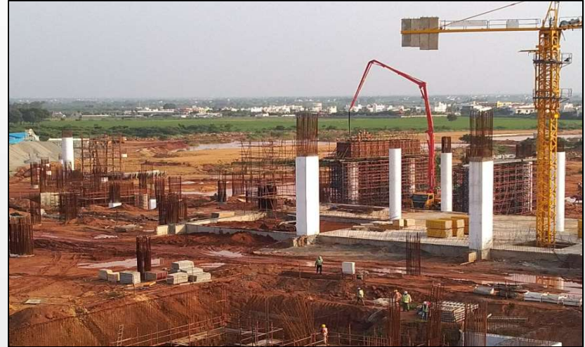
Trichy Airport Modernization - In Progress
