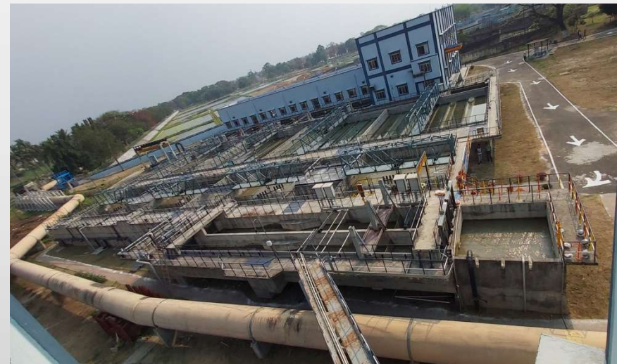
Palta WTP, West Bengal
