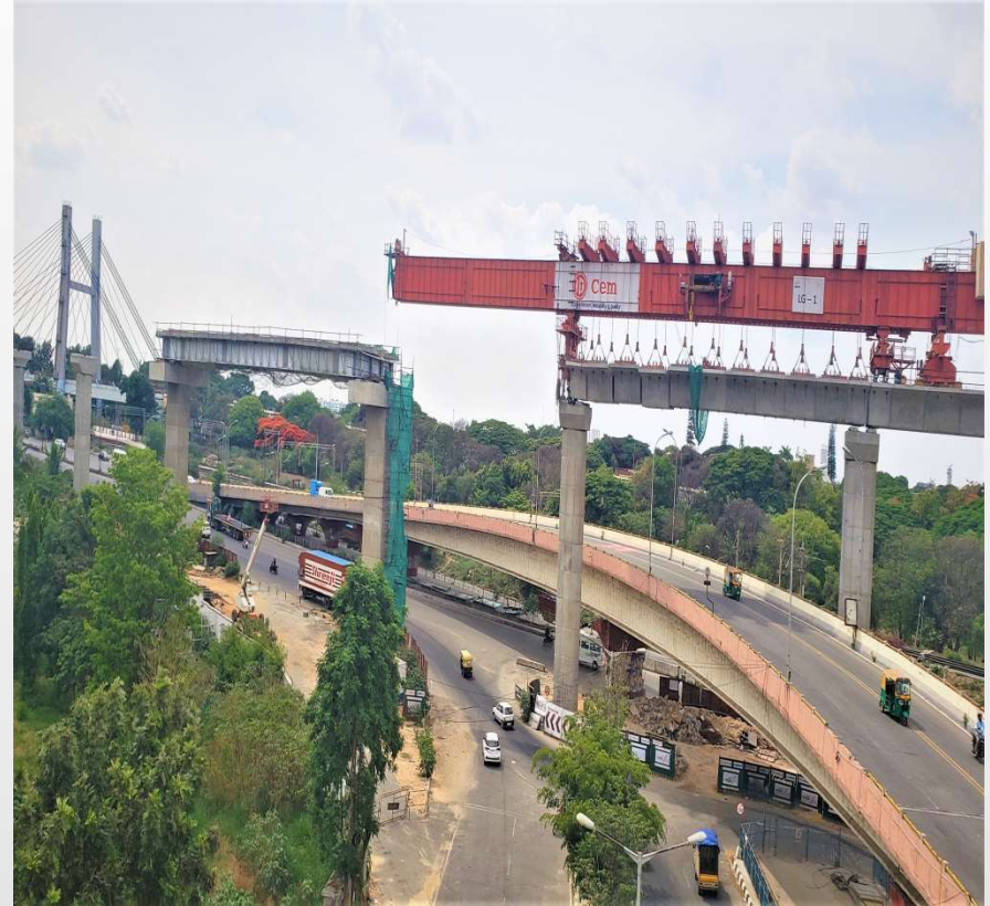
LG Crossing Over Existing Flyover, BMRCL Project
