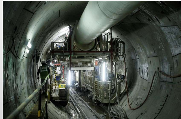
TBM Tunnel, Mumbai Metro
