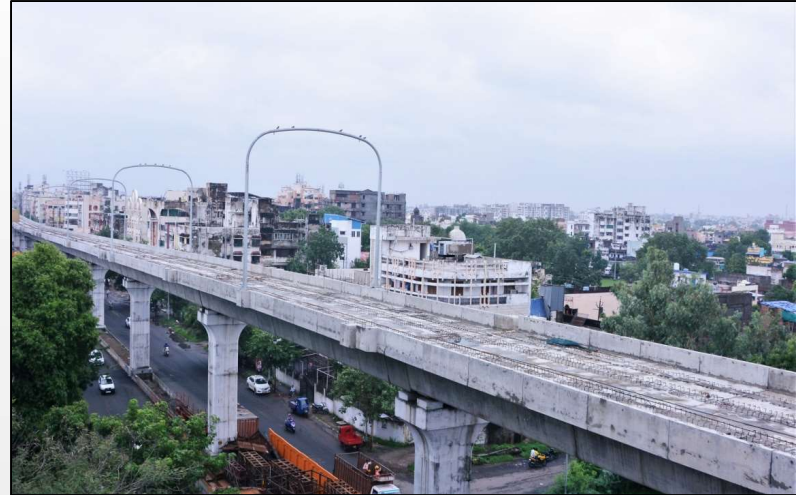
Nagpur Metro Viaduct
