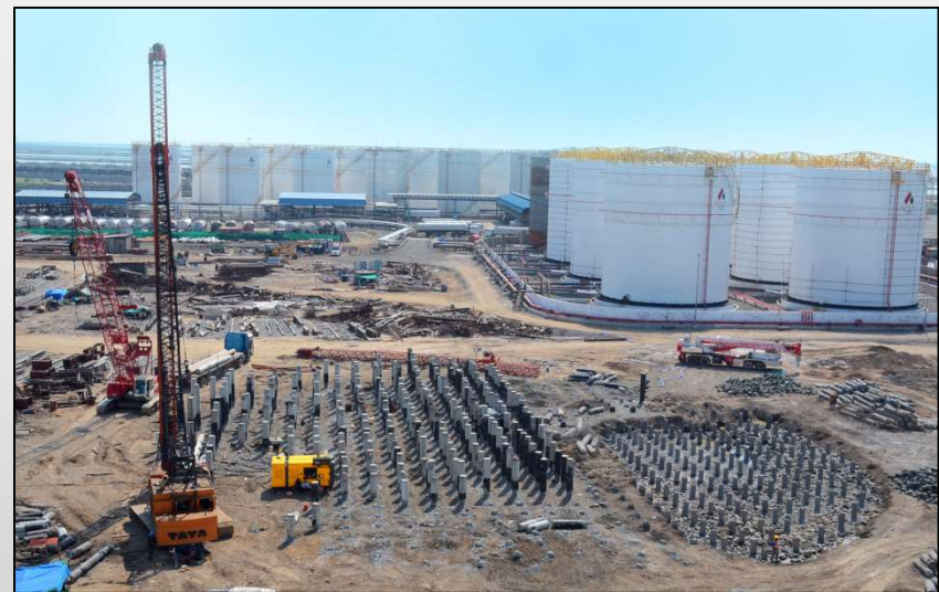
AEGIS Kandla, Precast Piling Project
