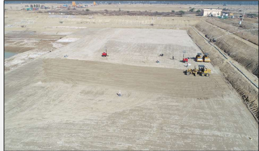
Ground Stabilisation work for Nuclear Power Corporation
