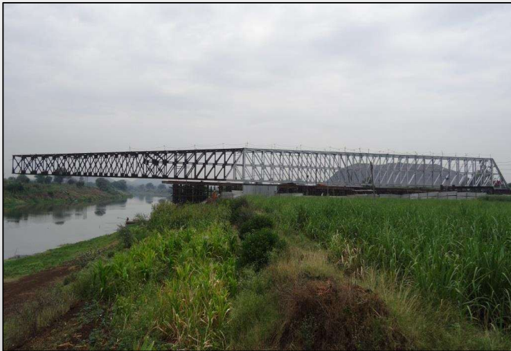
Dharna Bridge, Nashik
