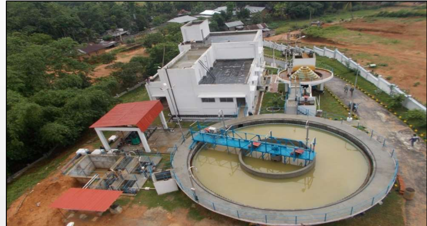
Agartala WTP project under Multilateral Funding
