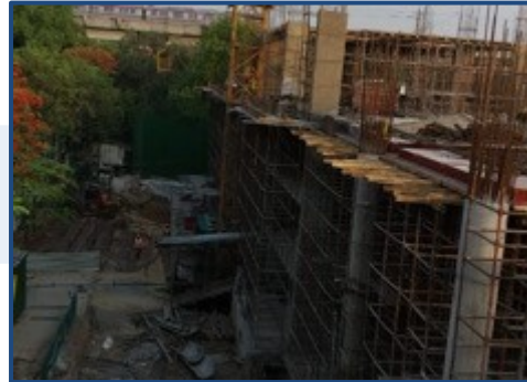
March 2019 Structure completed up to L3
