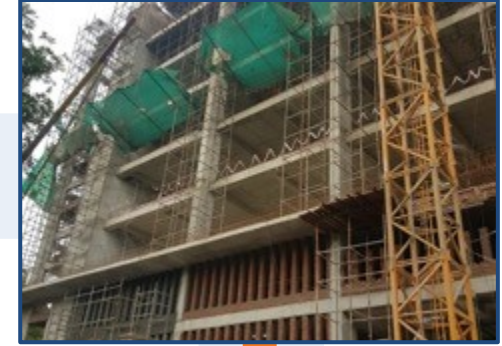
June 2019 Structure completed upto L6
