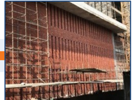
September 2019 Structure completed
