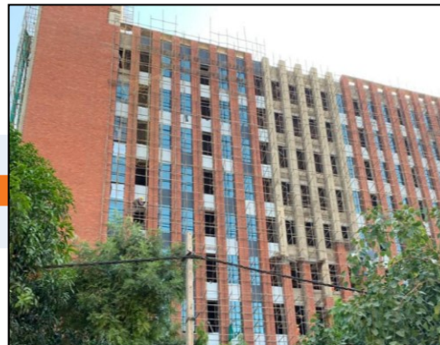
May 2020 Façade & Services installation
