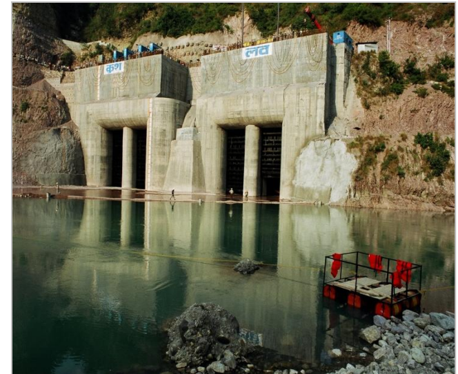
Kol Dam Project Client – NTPC Size – 7.5m X 14m X 115m
