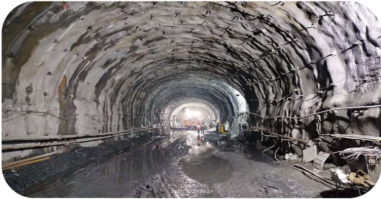
Sivok Rangpo railway tunnel project
