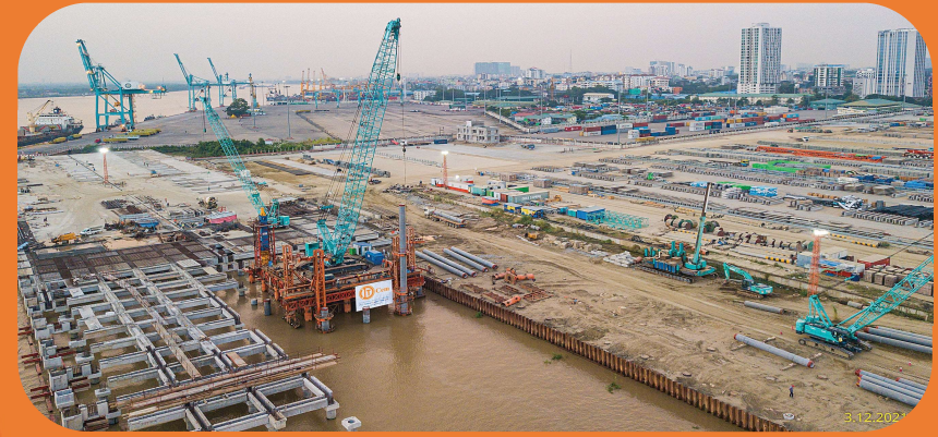
Container Terminal in Yangon International project, Myanmar
