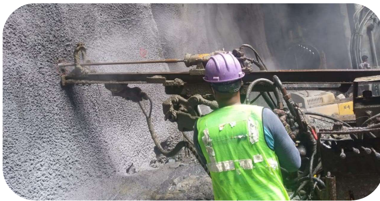
Rock bolt drilling in Mumbai UG station
