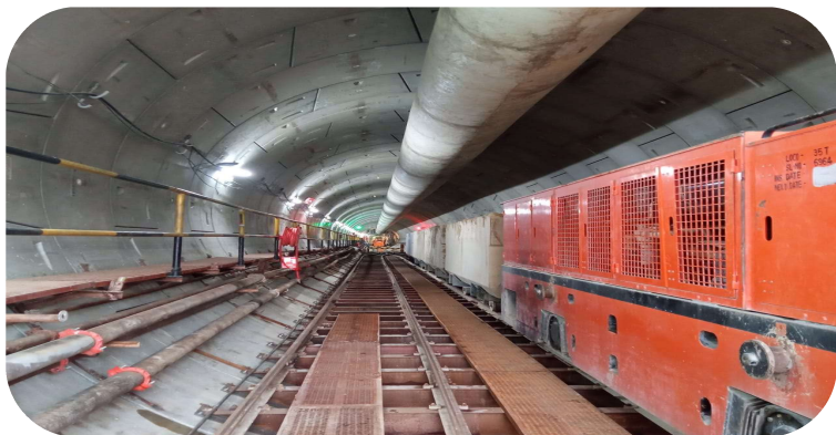
Bengaluru Underground Metro Project
