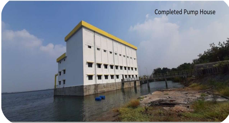
Water intake facility in Pune
