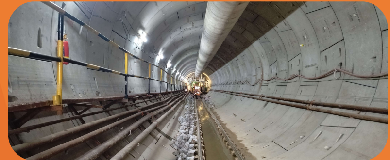
Bengaluru Underground Metro project
