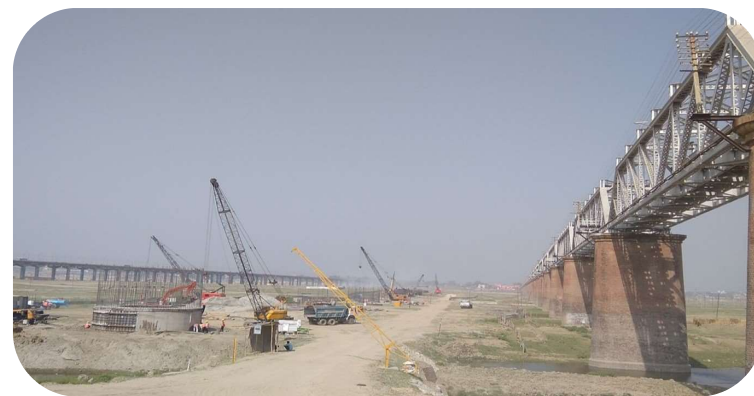
Ganga Steel bridge in Uttar Pradesh
