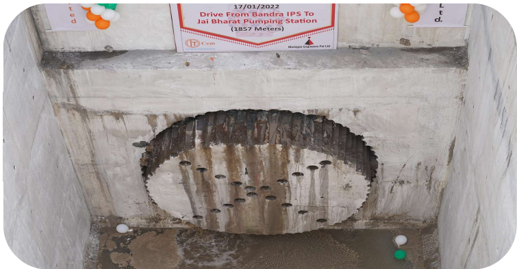
MCGM micro tunnel breakthrough in Mumbai
