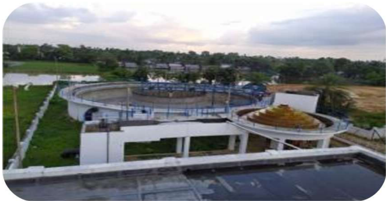
Water treatment project in Agartala, Tripura
