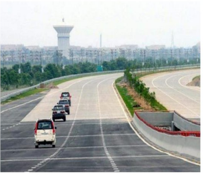
Crash Barrier at Yamuna Expressway
