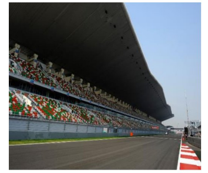
Grandstand Roofing at Buddh Int'l Circuit
