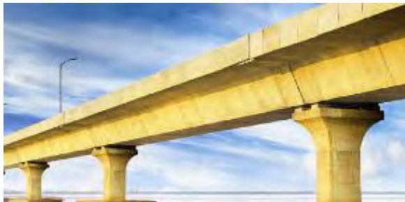
Dhola-Sadiya Bridge, Assam
