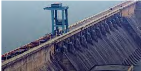
Hirakud Dam, Odisha
