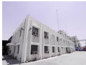
RFL I & II - Bahadurgarh
