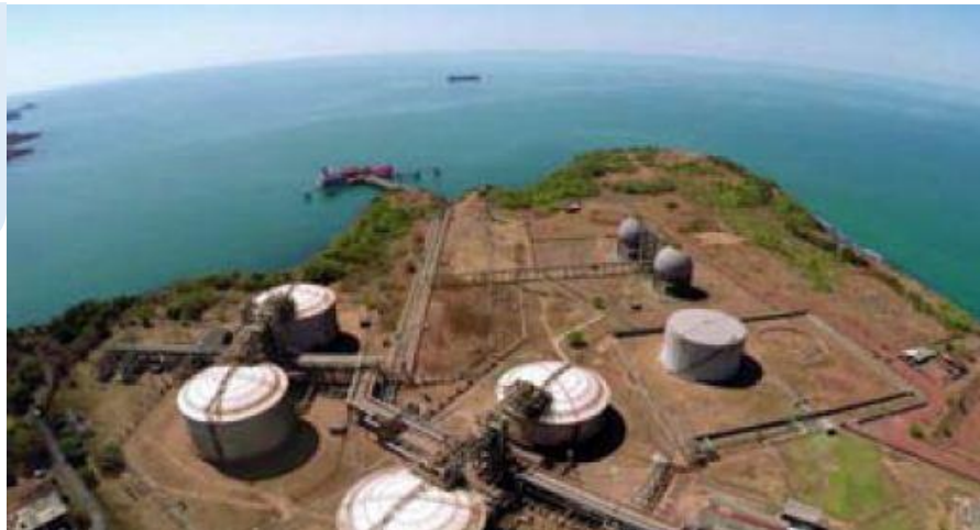
Storage tanks for raw material
