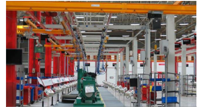
2010 - Parts Distribution Center , Phaltan
