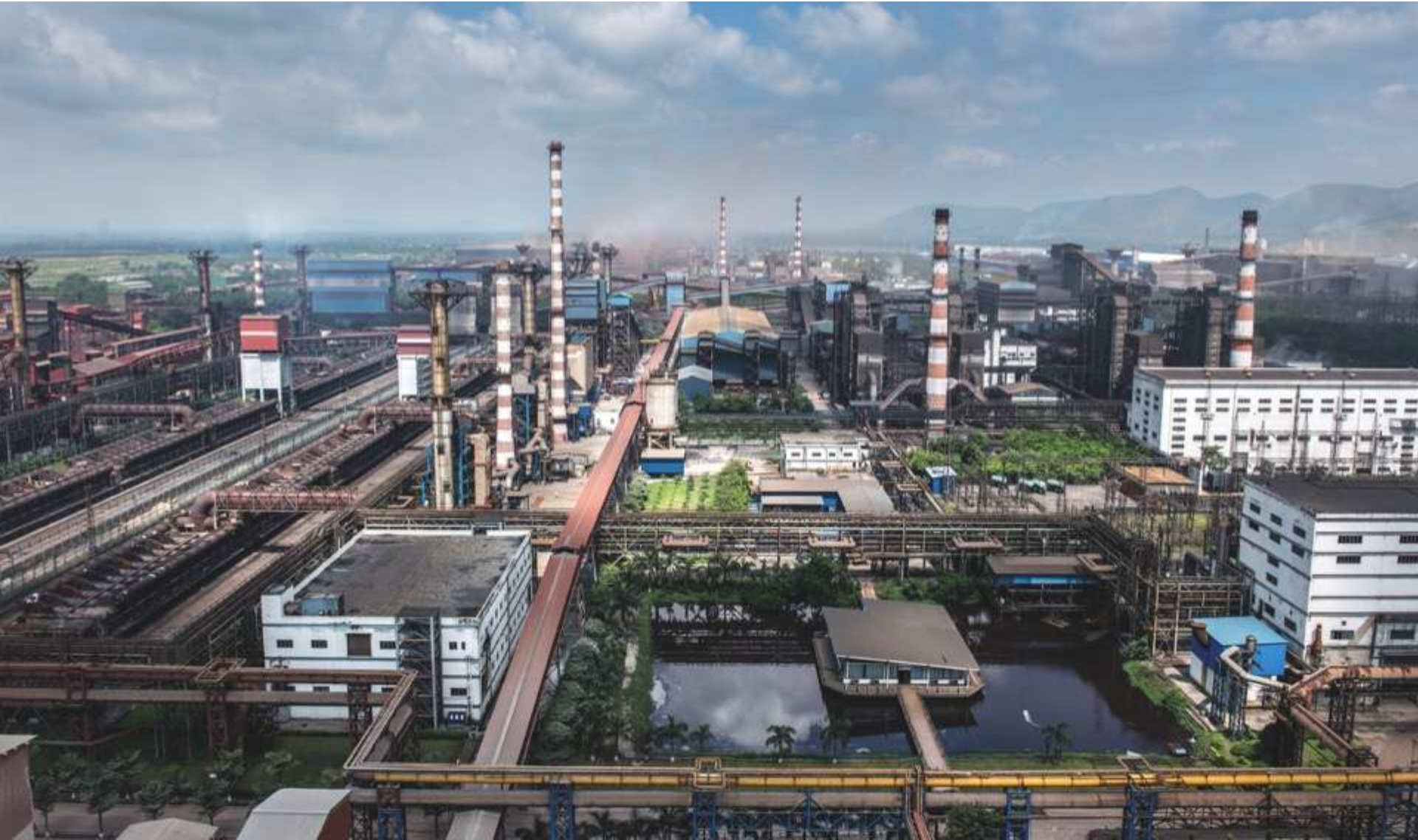
Aerial View of Raigarh Plant
