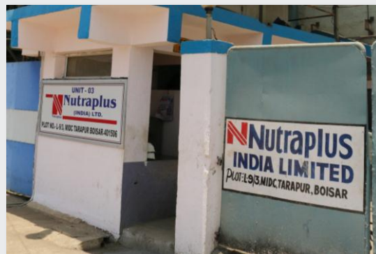
Unit 3 (Manufacturing Plant)
