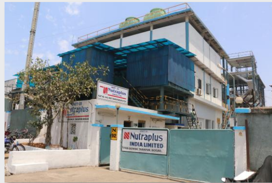
Unit 1 (Manufacturing Plant)
