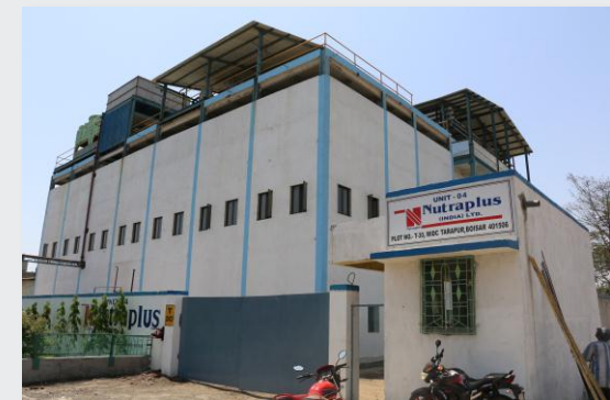
Unit 4 (Manufacturing Plant)
