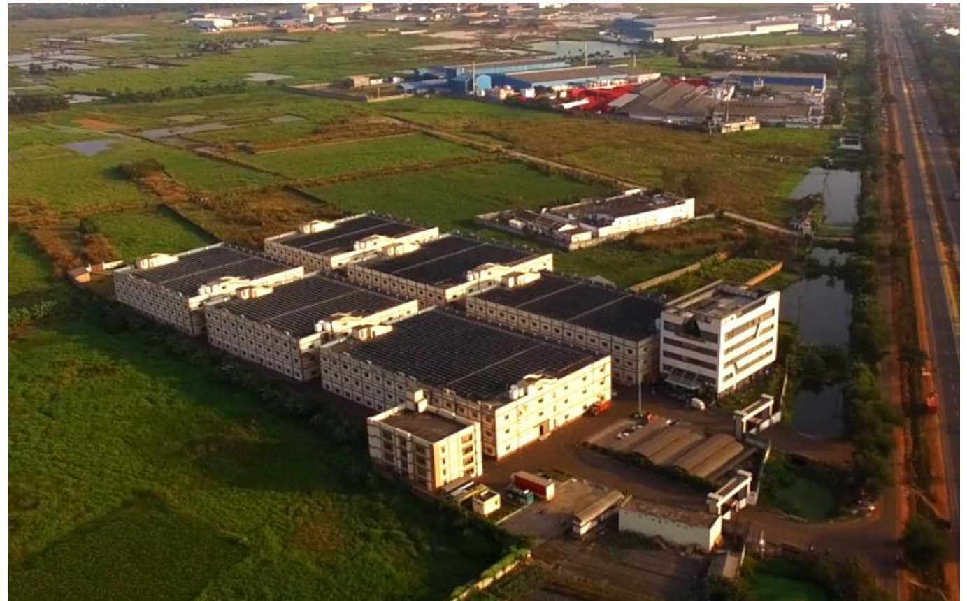
Rooftop solar power plant at Dankuni unit
