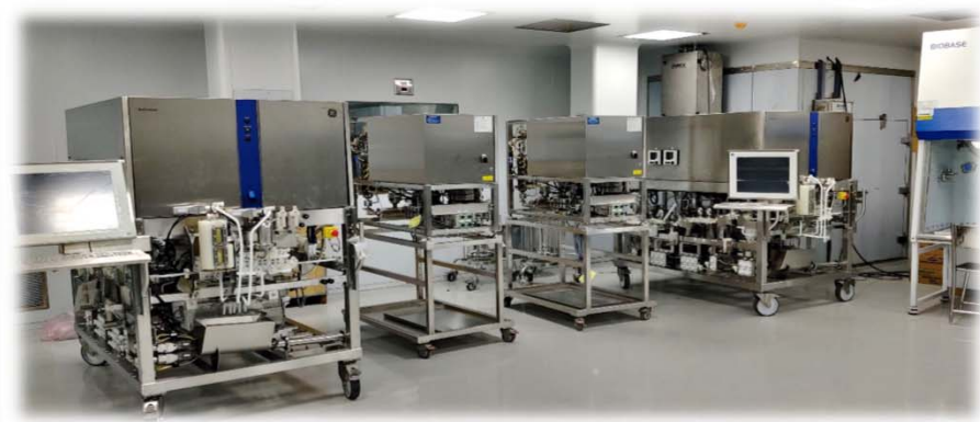
MAb purification suite - fully automated
