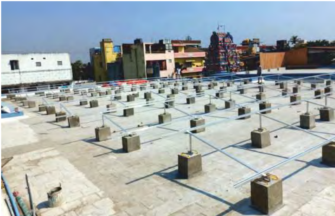
Installation of Solar Panel at Arulmigu Vadapalani Murugan Temple, Chennai
