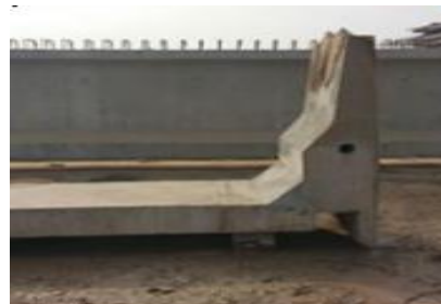
Fabricated Casting Panels and Moulds
