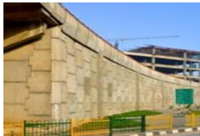
Reinforced Earth Walls
