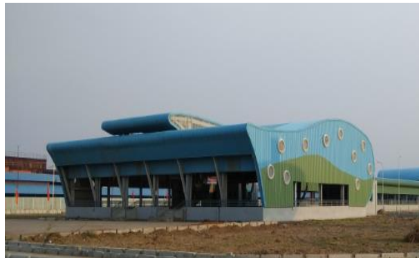
RO-RO Ferry Terminal – Dahej, Gujarat
