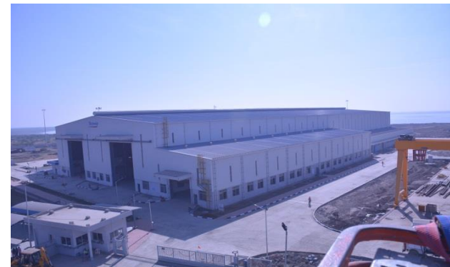
Technip – Dahej, Gujarat
