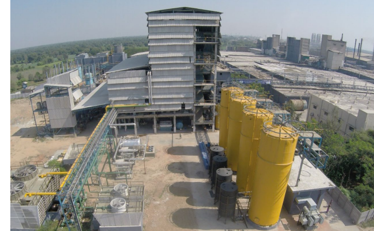
Multiple Effect Evaporator Plant (MEEP)
