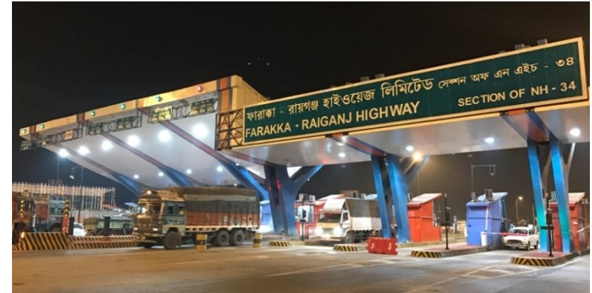
Farakka Raiganj Highway: Toll Plaza at Km 297
