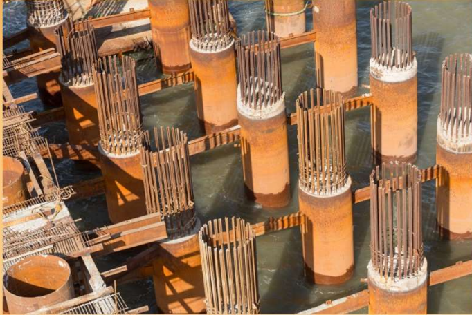
Marine Piling for Mumbai Port Project
