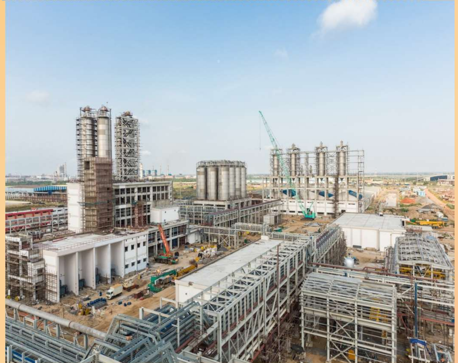
Construction of Industrial Project for Indian Oil Refinery, Paradip
