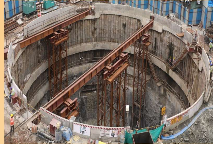
Diaphragm Walling at Mumbai Metro Line 3
