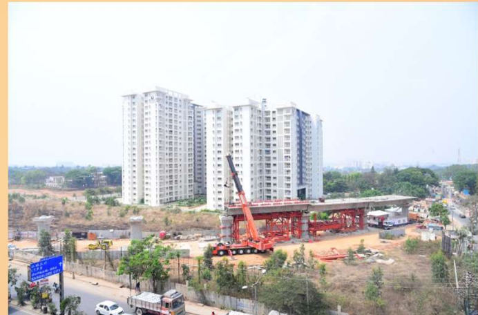
Bangalore Elevated Metro Project
