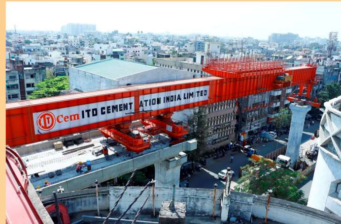
Nagpur Metro Elevated Project
