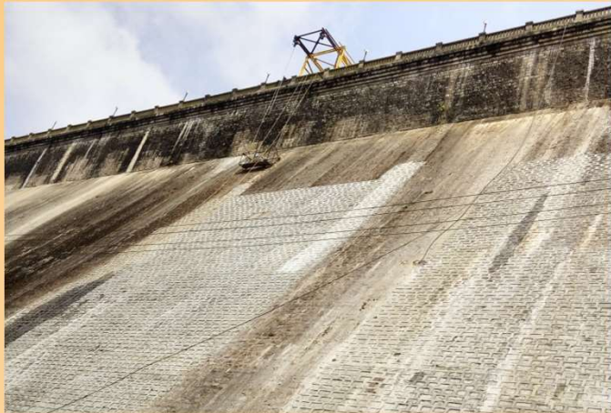
Karnataka Power Corporation – Dam Rehabilitation Project
