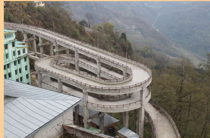
Piling & Civil Works for Gangtok Project
