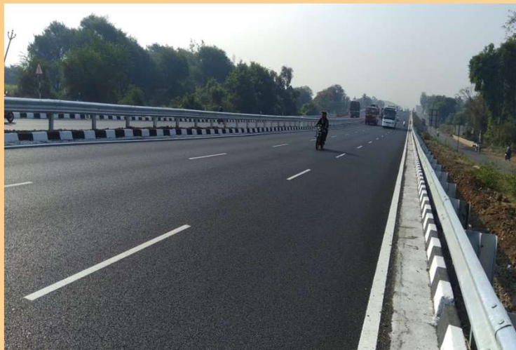
Pune Satara Road Project
