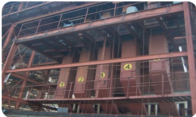
Bagasse Silos & Feeders of Boiler
