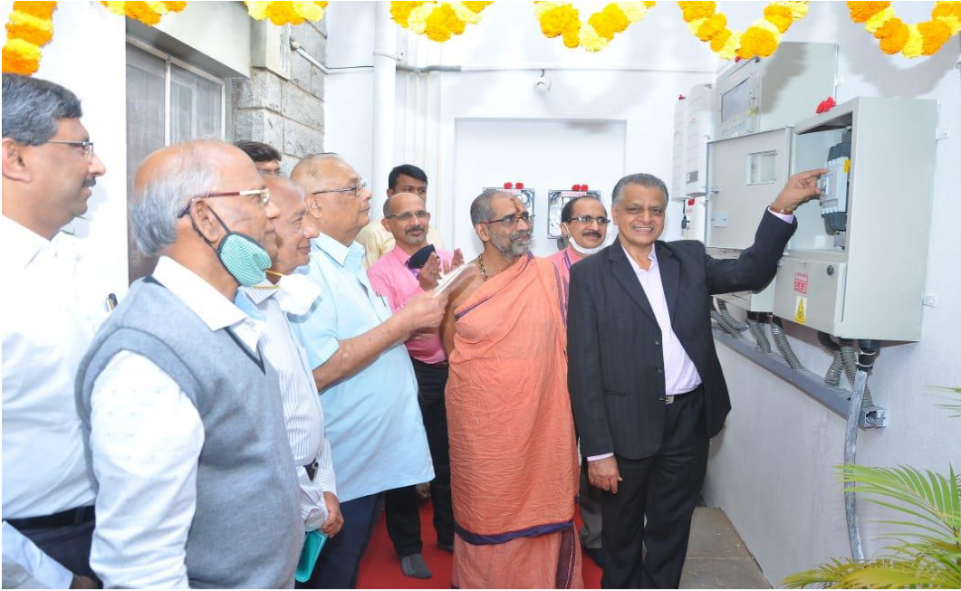
Solar roof-top photovoltaic system installed at the campus of Poornaprajna Institute of Scientific Research, Devanahalli, Bengaluru.
