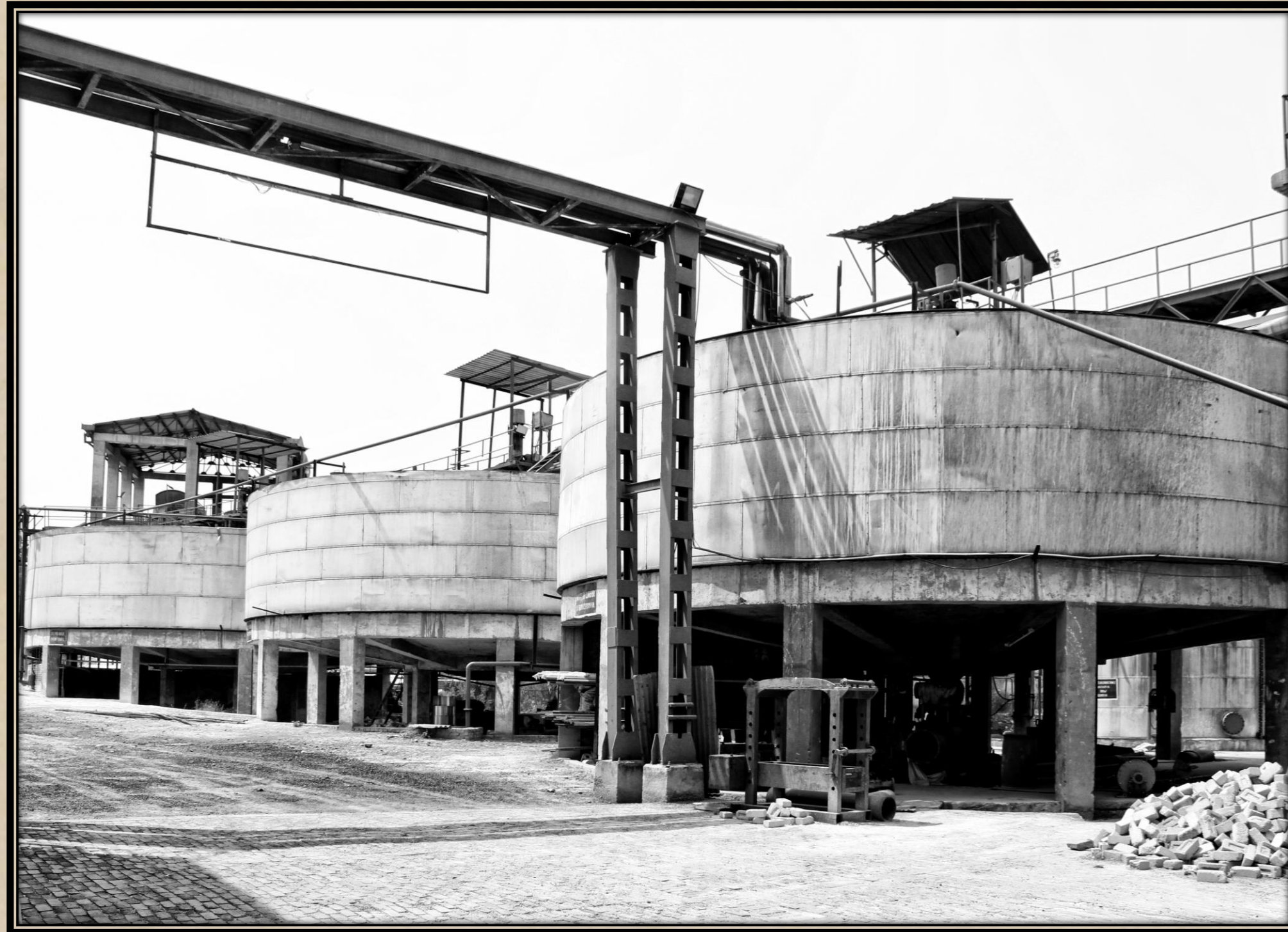
Chemical Recovery Plant - Conventional Recovery system with 2.5 MW turbine running independently on Recovery boiler steam.
