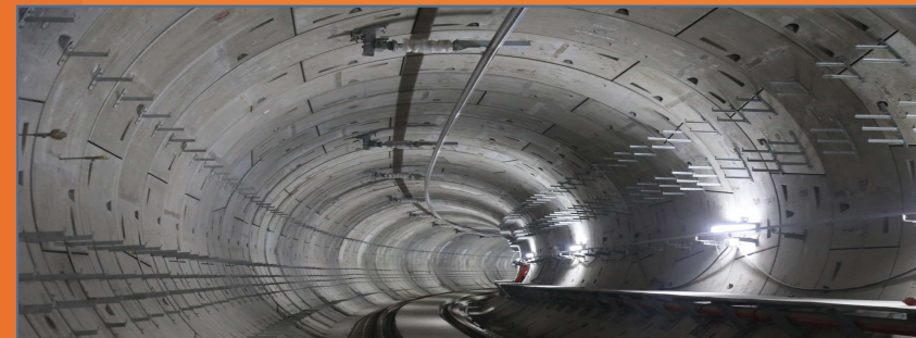
Mumbai Metro underground tunnel in Maharashtra
