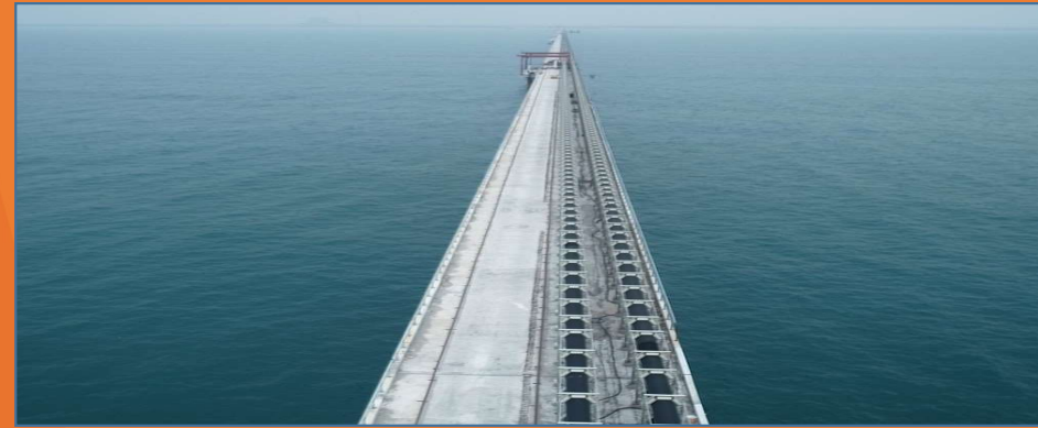
Udangudi approach trestle marine works in Tamil Nadu
