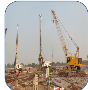
FOUNDATION AND SPECIALIST ENGINEERING
