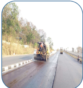
HIGHWAYS, BRIDGES AND FLYOVERS
