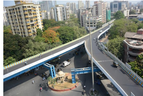
Meenatai Thakre Flyover
