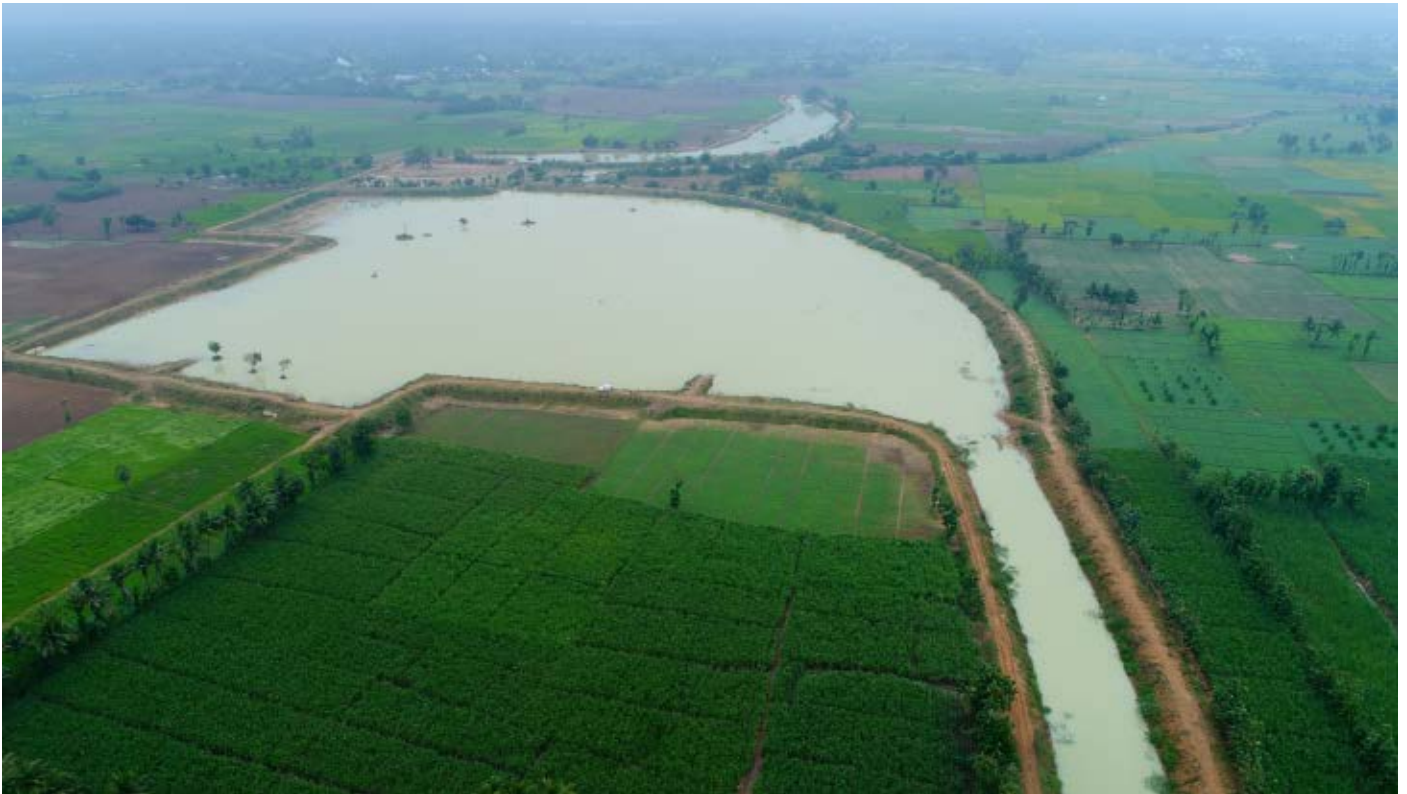
Desilting of Ellappanpettai Eri
