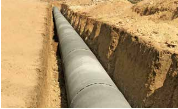
1700 mm dia PCCP pipeline laying for KPCL Bellary Thermal Power Plant, in Karnataka
