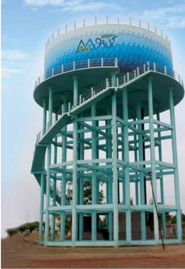
1000 KL Capacity Overhead Service Reservoir for Raipur Water Supply Scheme, in Chhatisgarh.
