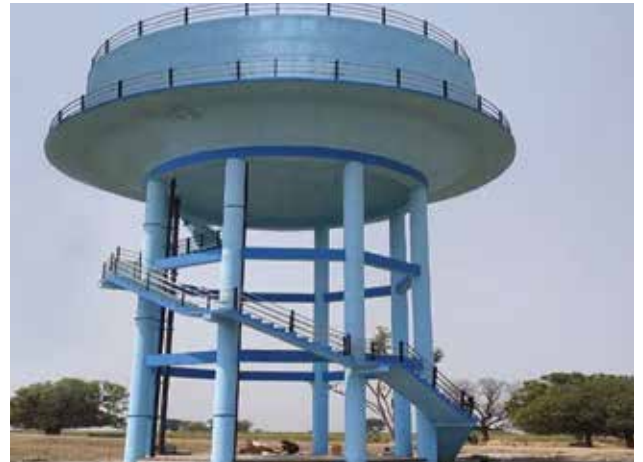
410 KL Capacity Overhead Service Reservoir for Kandaila Multi Village Rural Water Sully Scheme in Rewa Dist., in Madhya Pradesh.
