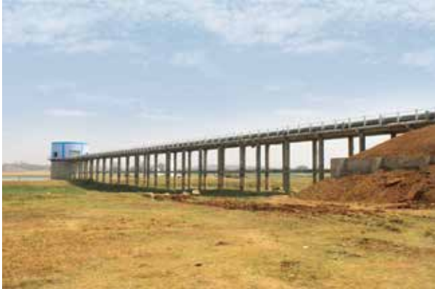
35.90 Intake Well 35.90 MLD ( 10 mtr dia 17 mtr deep) at Jhal Village for Indwar Multi village Rural water Supply Scheme, in Madhya Pradesh.
