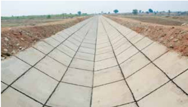
Canal Lining for Asolamendha Project Renovation Division, Gowardhan Branch, in Maharashtra.
