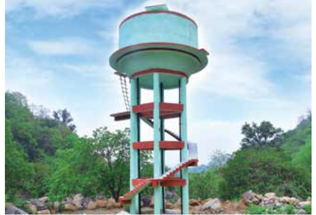
120 KL Overhead Tank 12 Mtr Staging at Gajapati for Gajapati Water Supply Scheme, in Odisha.
