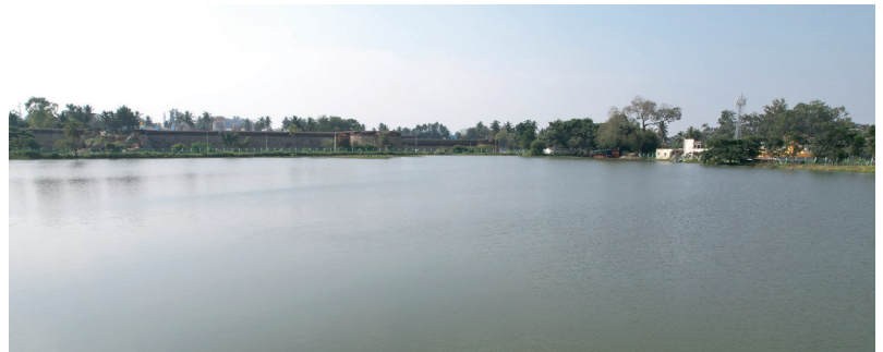
Our Team concluded the Devanahalli Lake restoration project in partnership with United Way India. The project spans nearly 17 acres of land, and the lake itself has a capacity of over 535 million liters of water. This initiative is expected to raise the groundwater table and improve the moisture content in the soil, benefiting up to 5,000 people living in and around the area
