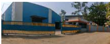
Khopoli, Maharashtra Installed capacity of 80,000 MTPA
