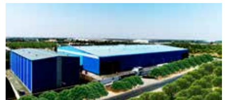
Sanand, Gujarat Installed capacity of 1,25,000 MTPA
