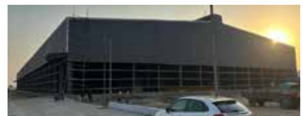
Sanand, Phase-II, Gujarat Proposed capacity of 1,70,000 MTPA
