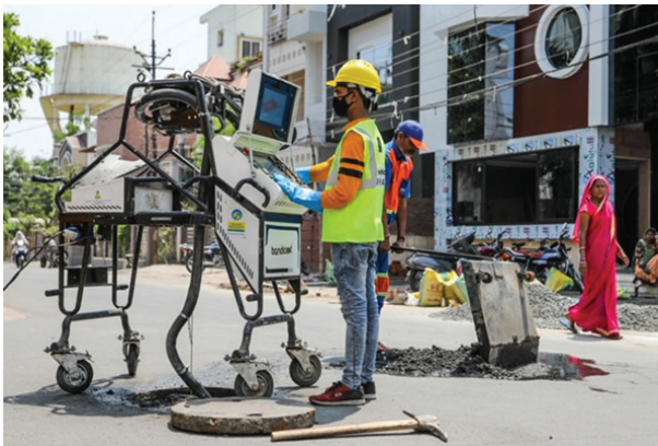
Bandicoot Robotic Manhole Cleaning Machine
