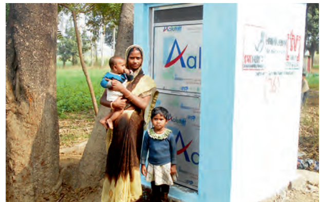
➤ Ms. Asha with her children in front of her newly constructed a toilet in village Sarhara, Hallia Block, Mirzapur district, Uttar Pradesh
