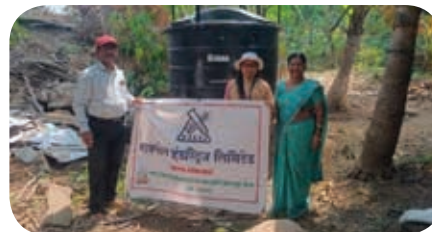
Bio Gas Unit – Amdoshi, Taluka Roha, Raigad
