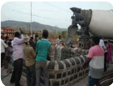
Repairs of water wells at Talaghar, Roha, Raigad
