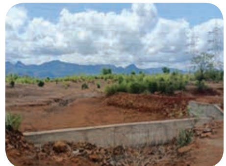
Desilting of River at Kudali, Atone
