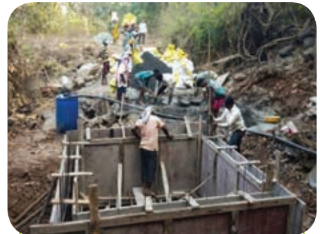
New water tank construction at Pale Khurd Adivasiwadi Village, Raigad
