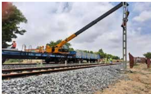
RE work in progress
