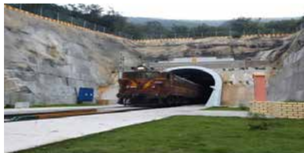
Tunnel on KRCL Line
