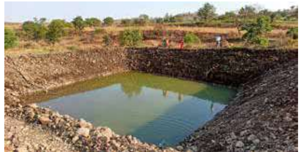
Water harvesting structures
