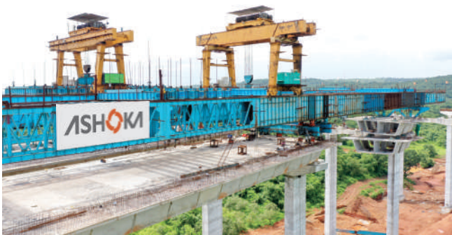
Mopa Airport Link Road
